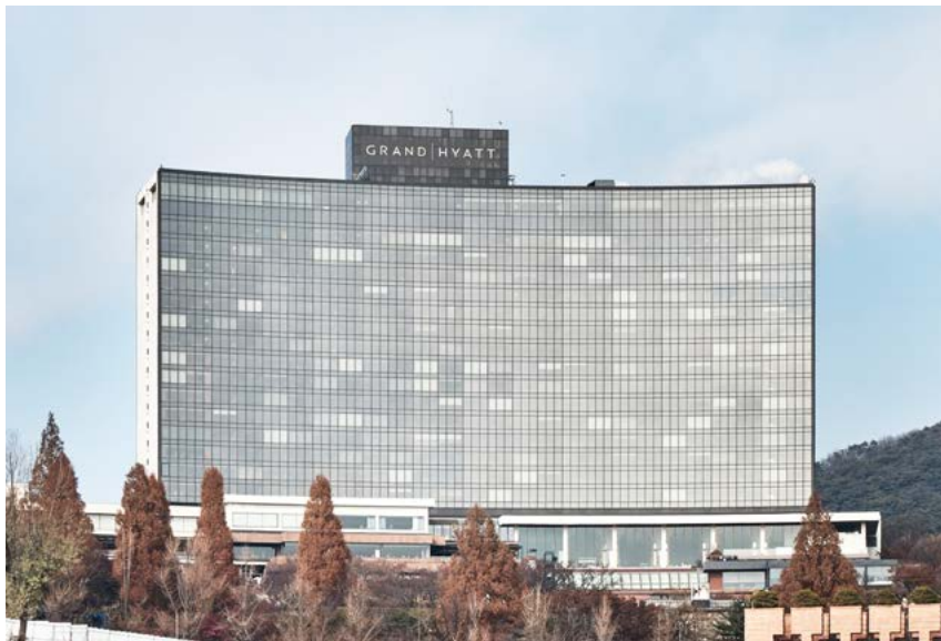
Grand Hyatt Seoul 4 units x 240m/min elevators
