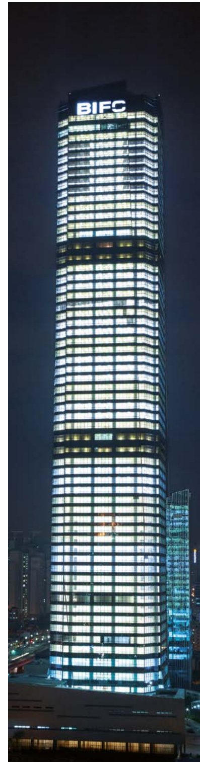
Busan International Finance Center 2 units x 600m/min elevators (the fastest in Korea), 3 units x 540m/min elevators, 8 units x 480m/min elevators and 6 units x 360m/min elevators (32 in total), 14 escalators
