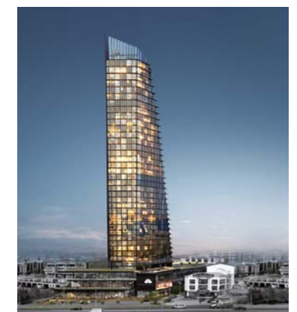
Türkiye Inanlar Terrace Lotus 5 units x 150m/min elevators (12 in total), 4 escalators
