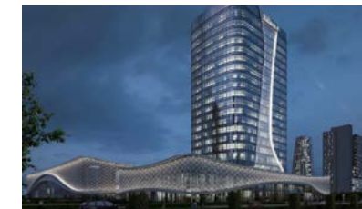
Uzbekistan IBC Hotel 10 units x 150m/min elevators (19 in total)
