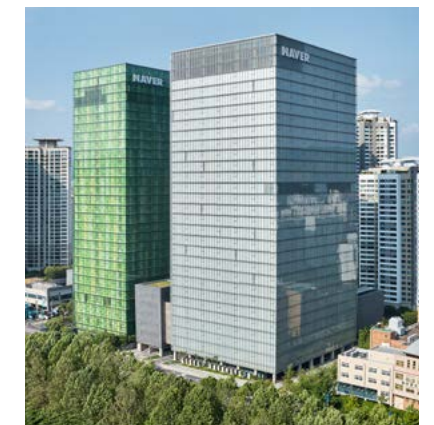
NAVER 1784 (New corporate headquarters) 10 units x 300m/min elevators, 10 units x 240m/min elevators (20 in total). The world's first robot-friendly building. Features a 'Roboport', an elevator dedicated to robots, Linked Rookie, the self-driving service robot, and passenger elevators
