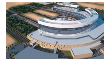
Saudi Arabia Security Forces Medical City 21 units x 150m/min elevators, 38 units x 105m/min elevators (184 in total), 24 escalators
