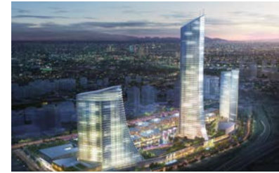
Türkiye Metropol Istanbul 6 units x 360m/min elevators, 1 unit x 300m/min elevator and 26 units x 240m/min (93 in total), 26 escalators
