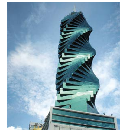
Panama F&F Tower 5 units x 240m/min elevators
