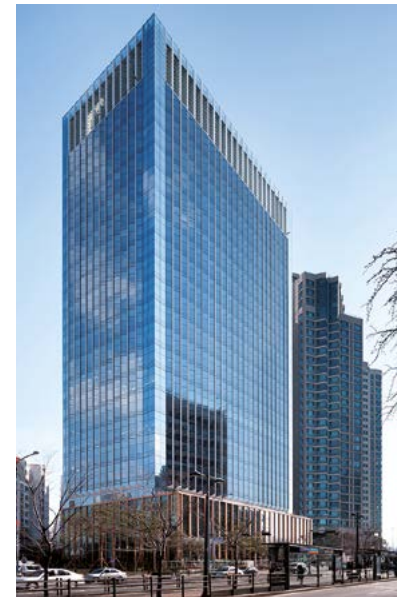
LG U+ Yongsan Office Building 2 units x 240m/min double deck elevators (the first in Korea), 4 units x 240m/min elevators and 2 units x 210m/min elevators (10 in total), 2 escalators
