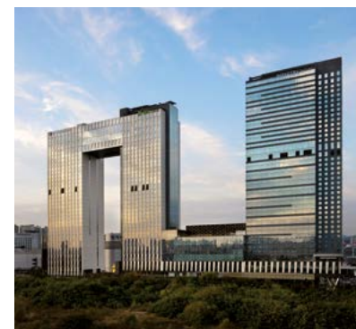
Seoul Dragon City 23 units x 240m/min elevators, 4 units x 210m/min elevators (33 in total), 10 escalators
