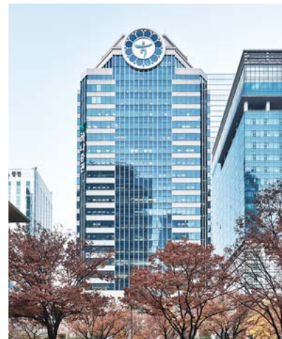
Main Building of HANA Financial Investment 8 units x 240m/min elevators, 1 unit x 120m/min elevator and 2 units x 90m/min elevators (11 in total)
