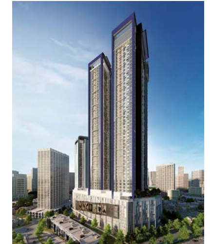
Malaysia Space Residency (Vistana Tropika) 6 units x 300m/min elevators, 4 units x 240m/min elevators and 3 units x 210m/min elevators (23 in total), 2 escalators
